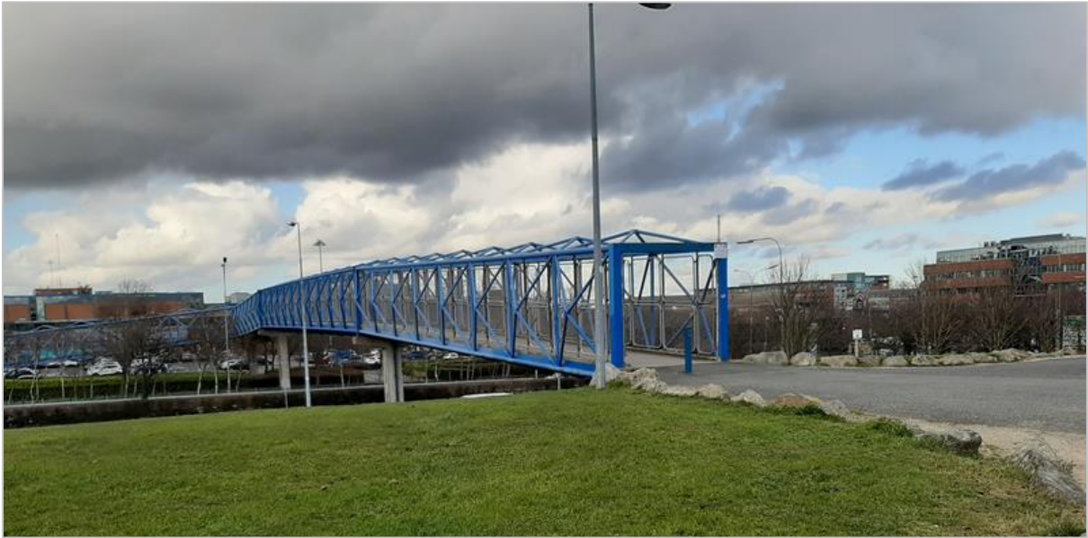
Figure 2-11 Pedestrian Footbridge over the N81 Dual Carriageway
