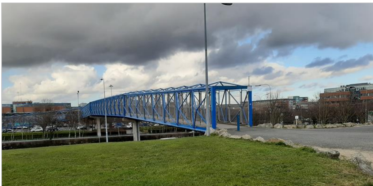
Figure 3-11 Pedestrian Footbridge over the N81 Dual Carriageway
