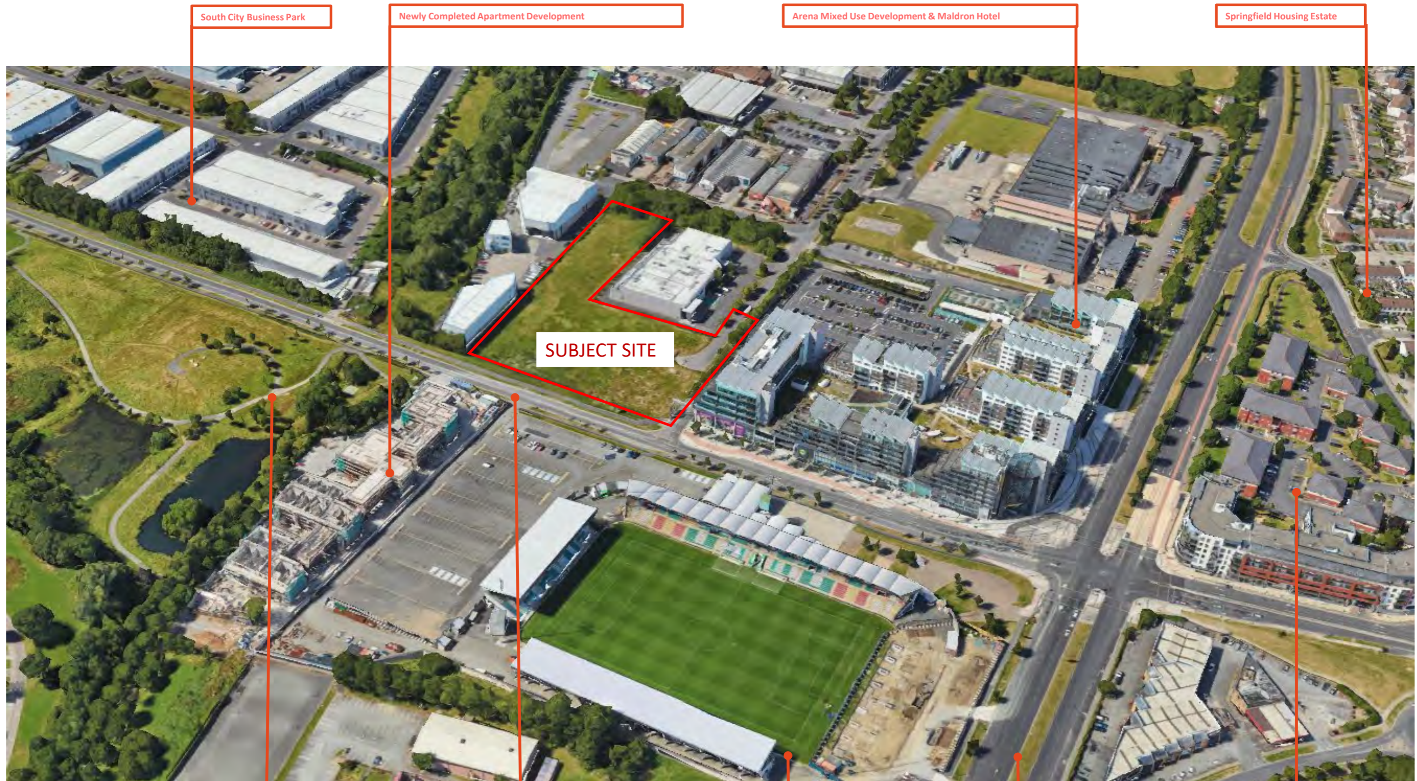
Aerial View to South West
