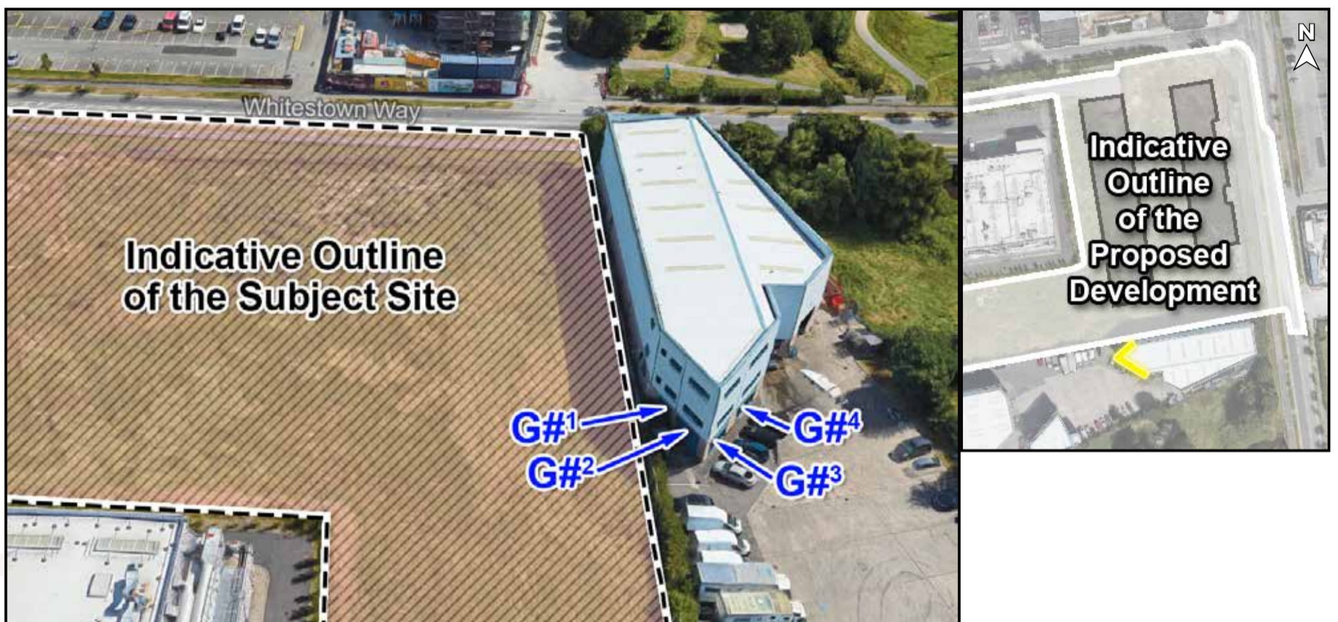
Figure 3.8: Highlighted areas indicate the position of assessed windows (L), Aerial view of assessed location (R)
