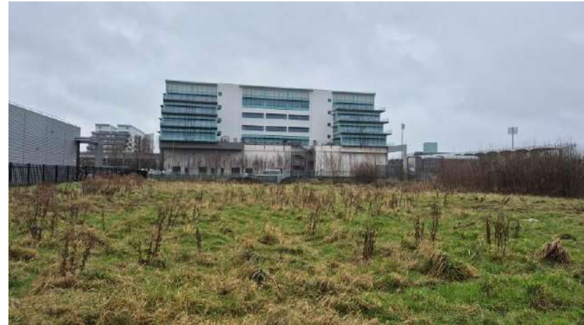
Plate 2: Northern part of site, facing north towards the site entrance
