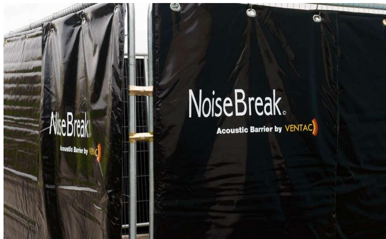
Figure 17: Temporary Construction Noise Barrier © Ventac
